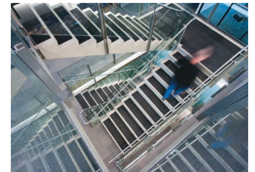
"Rather than treating the stair merely as a functional component, the team worked together to make it the centrepiece of the building's interior," says Kelly McCardle
